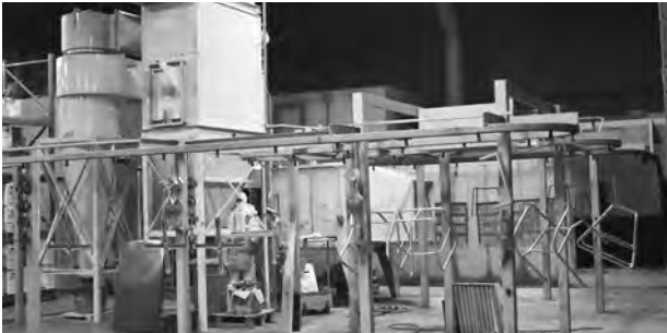
In-house Conveyorized Powder Coat application center
